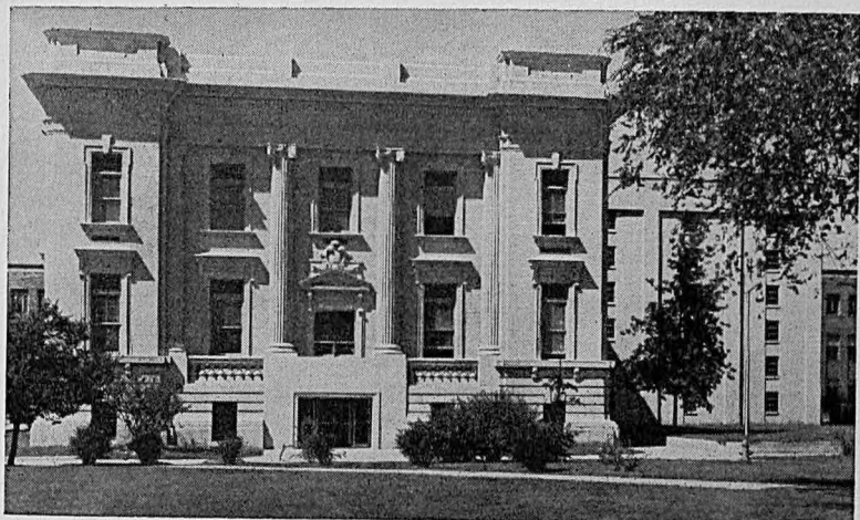
The Indiana State Teachers College Library was remodeled, and a new wing was added in 1957.
