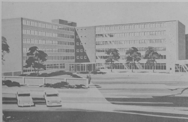
The new women's residence to be opened in Fall of 1959, is shown above. The building provides housing for 300 women students.
