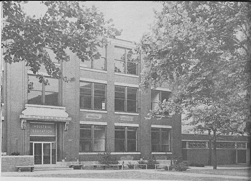
Industrial Education Building was completely remodeled and re-equipped in 1957.
