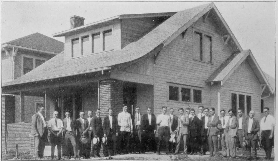
Another view of the above house made ready for plastering at the end of five weeks summer session.
