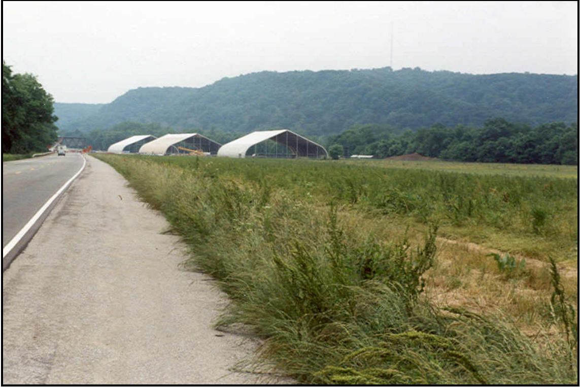
Figure 1.11. The Knob Creek site from the north--excavation structures above the 300, 200, and 100 Blocks, Knob Creek beyond treeline to the right and Ohio River beyond treeline to left.
